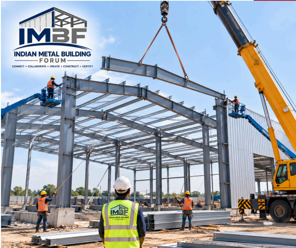
Industrialized metal building construction
