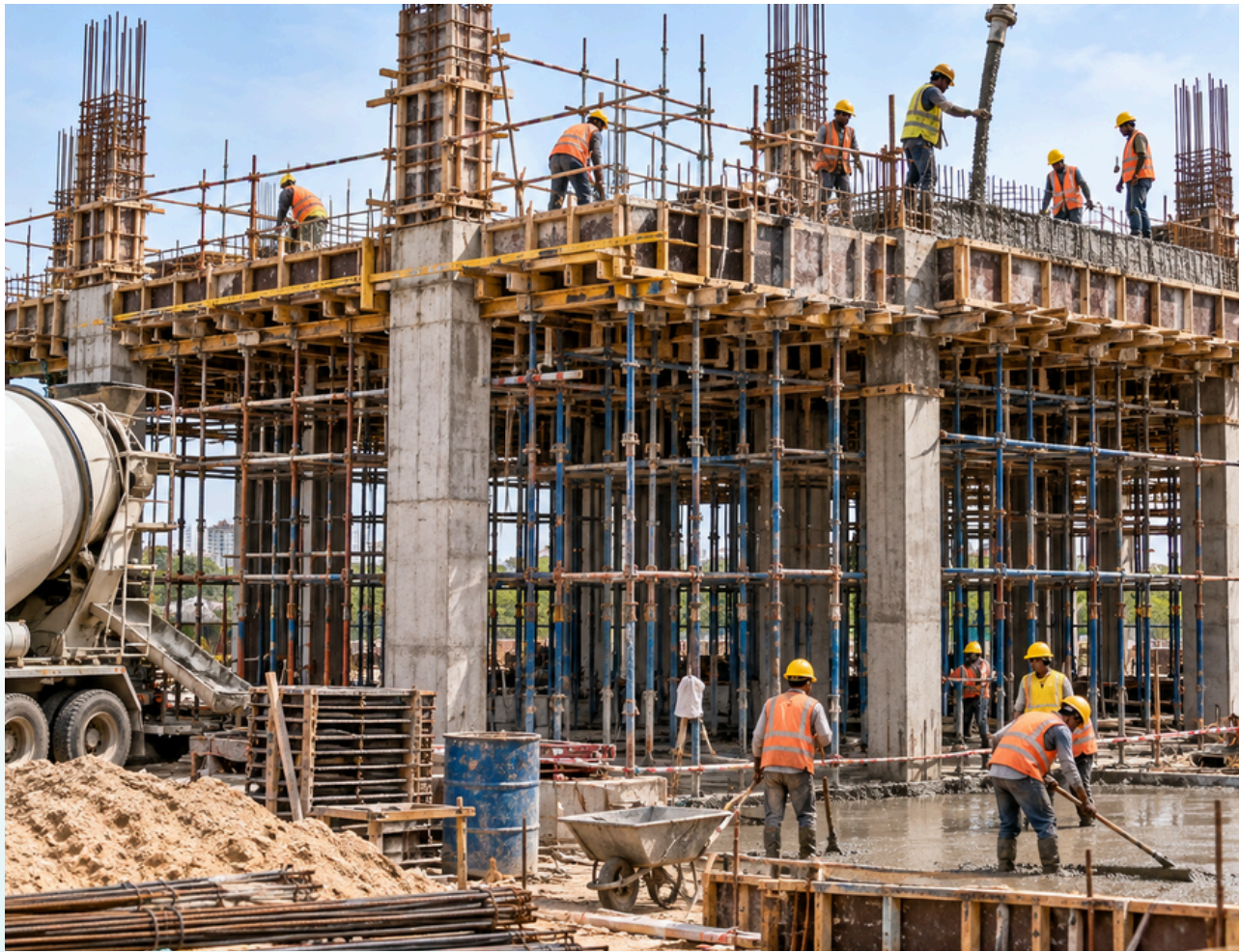
Traditional site construction
